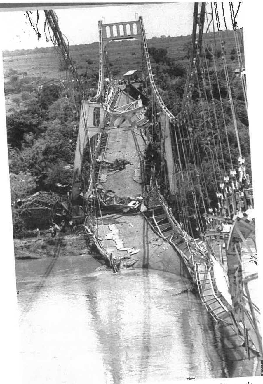
A casualty of El Salvador's civil war, the "Golden Bridge" was destroyed in an early-morning guerrilla attack.
